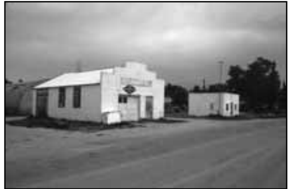
Service station, BN00-060
