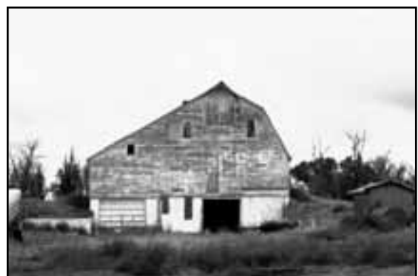
Gambrel roof barn with extended forebay, BN00-036
