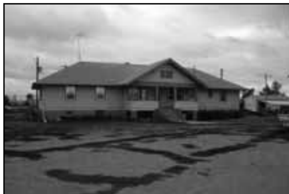
Former Harrisburg High School, BN01-009
