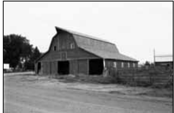
Example of gambrel roof barn, BN00-079
