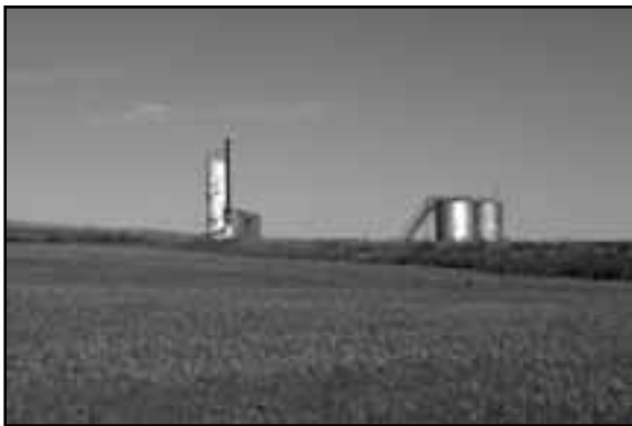
Oil heater and storage tanks
