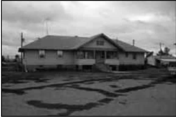
Former Harrisburg High School, BN01-009
