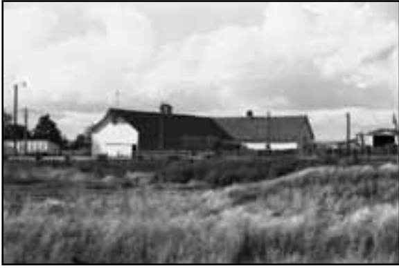
Gable roof barn with long narrow form located on Barrett Ranch, BN00-088
