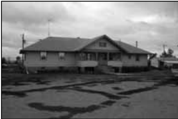
Former Harrisburg High School, BN01-009
