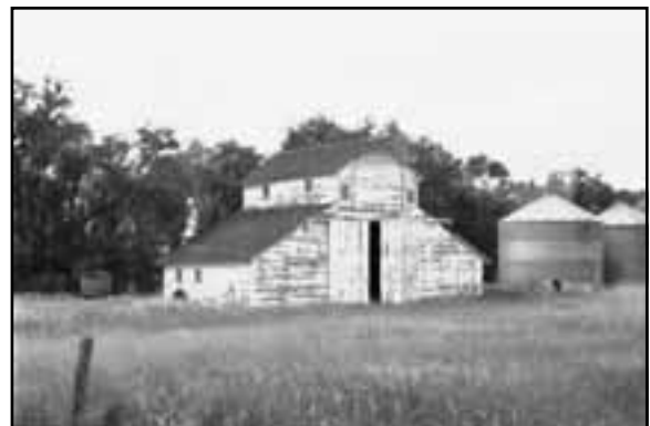
Example of monitor roof barn, BN00-085
